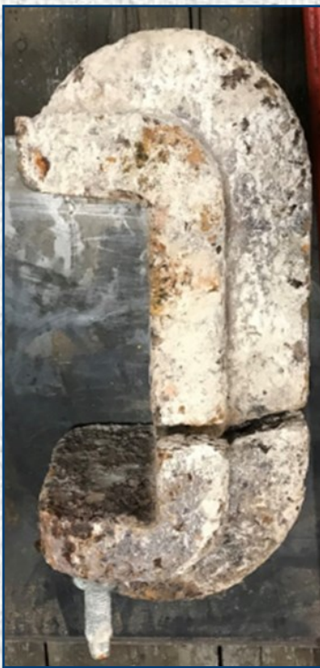
A broken top wedge required replacement.
