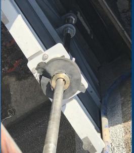
Lower bellows shield the operator stem below the hoist.
