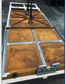
New gates prior to installation and painting. New patterns and castings were required for the upper and lower ductile iron leaf discs to have the same look as the original gates installed in 1905.
