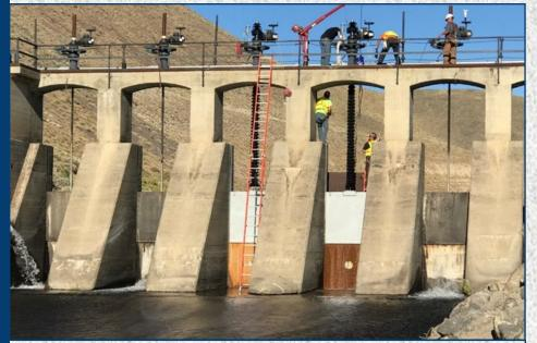
The downstream side of the two new leaf gates (third and fourth from left) after installation.
