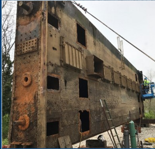
Kaighn Avenue Tidal Dam West Tide Gate before (above) and after (below) repairs and recoating.
