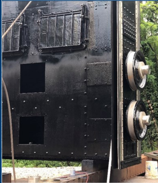
Kaighn Avenue Tidal Dam West Tide Gate before (above) and after (below) repairs and recoating.
